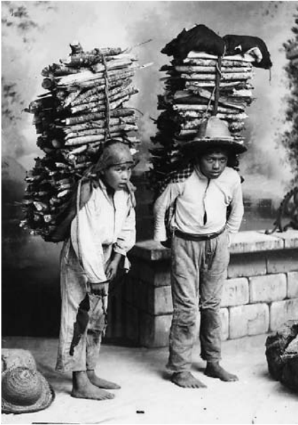
Figure 6. "Beasts of Burden, poor and lamentable pariahs."
